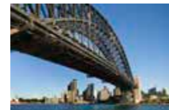
Corrosion protection coatings in harsh environments
